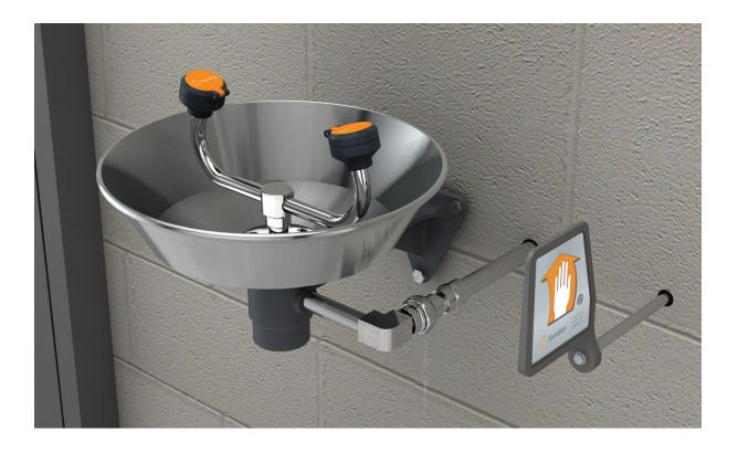
Application: Freeze-resistant eyewash for wall mounting. Valve and supply line are located behind wall in heated area to prevent freezing. Self-draining valve permits water to drain completely from unit after use. Since unit is intended for use in cold weather conditions, consideration should be given to supplying unit with tempered water in accordance with ANSI Z358.1-2014. See "Tempering Units" section for more information.
